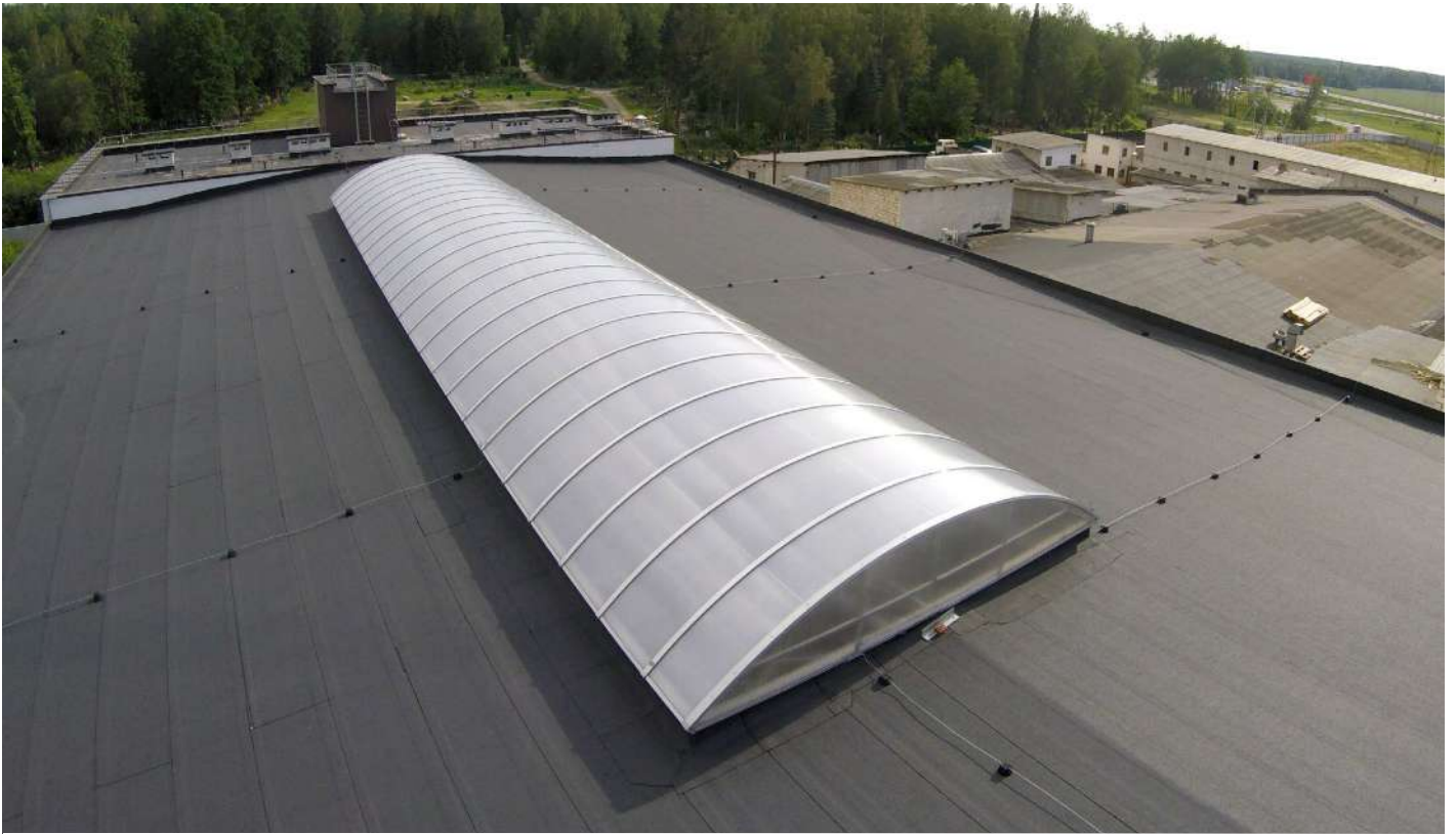
Gable ridge flat skylights on standard 1,5 x 12,0 m and translucent 6,0 x 12,0 m foundation with ventilating doors
