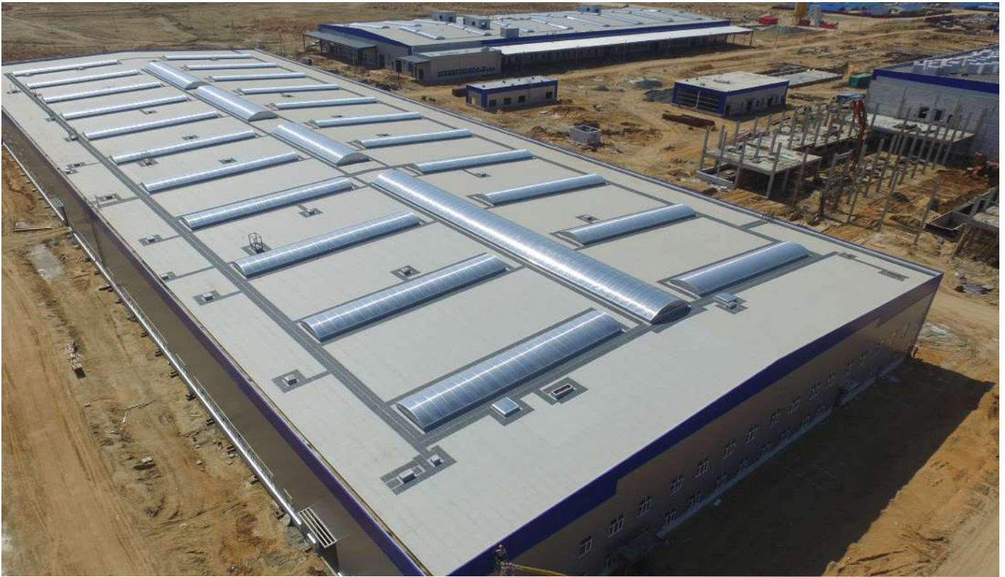
Gable ridge flat skylights 3,0 x 18,0 m, 4,0 x 18,0 m, 4,0 x 46,0 m (total area of the skylights is 6 516,5 sq.m.)
