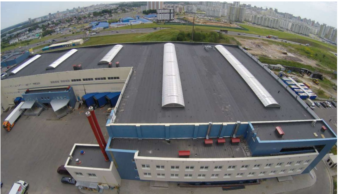
Gable ridge flat skylights 4,0 x 24,0 m with smoke extraction and ventilation doors
